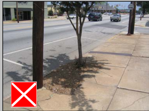
Neglected tree maintenance
