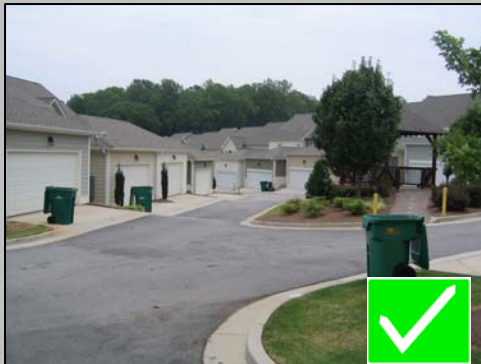
Rear alley in a new construction neighborhood
