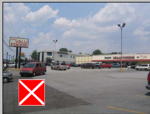
Inappropriate parking lot with parking between building and street, no landscaping
