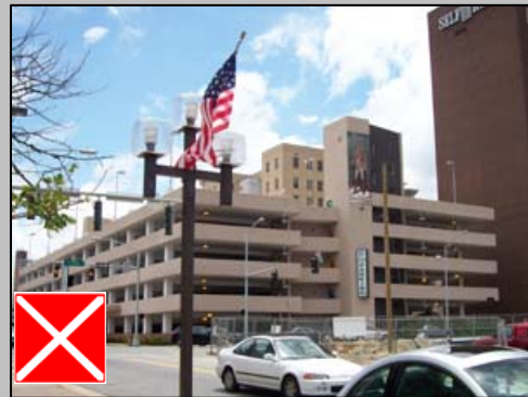
Decks that do not conceal automobiles and do not connect with the existing architectural style are not acceptable
