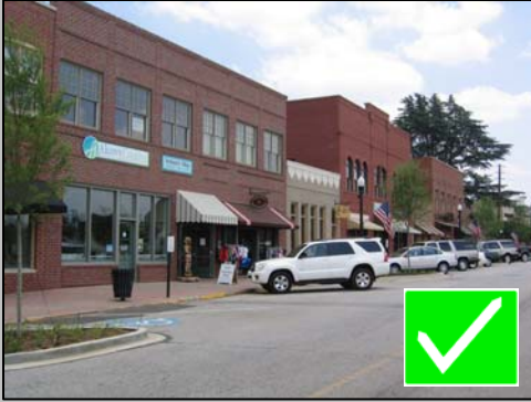
New development should emulate historic buildings of one and two stories
