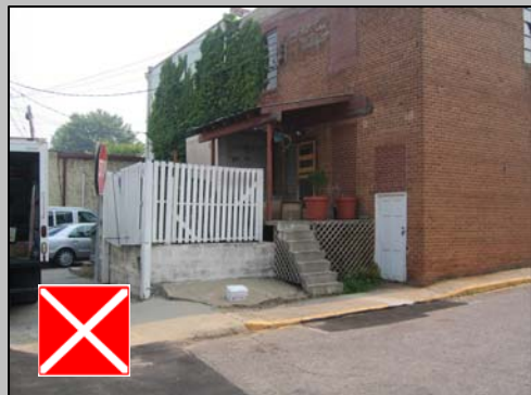
Buildings with unattractive rear entries do little to welcome pedestrians
