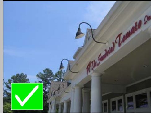
Gooseneck lighting fixtures
