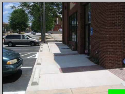
Sloped pavement toward store entrance
