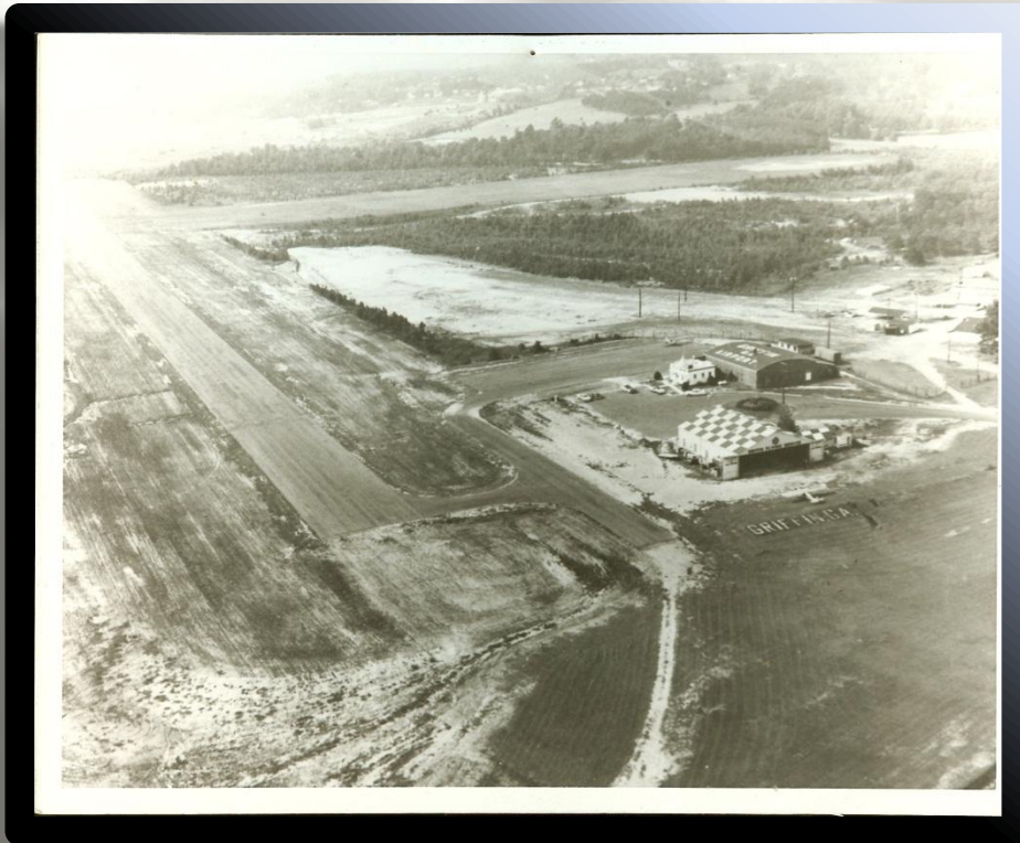
Year is 1955 – Griffin-Spalding Airport runway with paving completed
